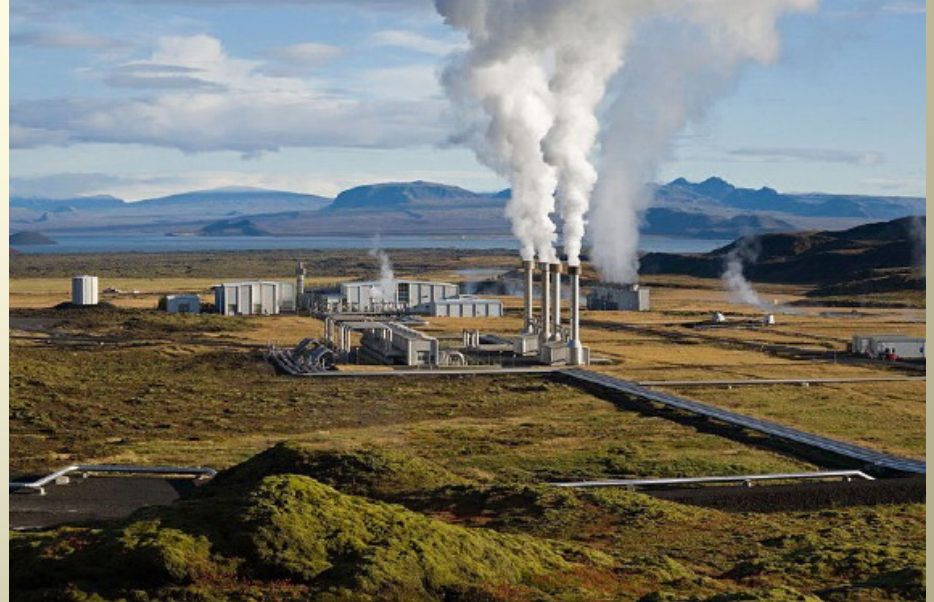
Nesjavellir Geothermal Power Plant (Iceland) Foto: Gretar Ívarsson
